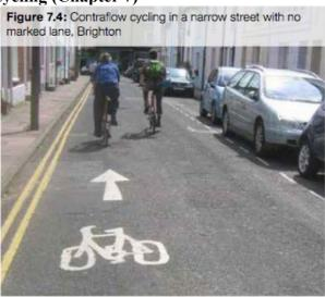
This should always be considered (para 7.3.4, p78). Contraflow cycling provides a more direct route for cyclists. On quiet low speed streets, there may be no need for a cycle lane. 'Where there is good visibility cyclists and on-coming drivers should be able to negotiate passage safely.'
