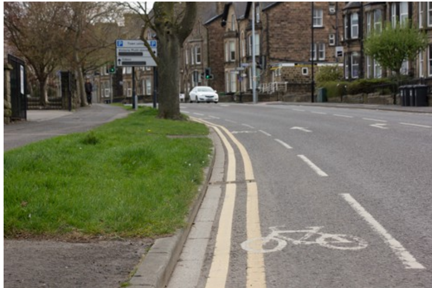
Illustration 7: Painted lane on East Parade (1m20, 30cm below the Absolute Minimum)
